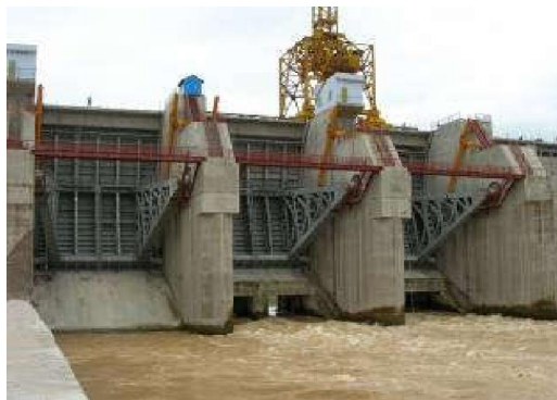
SeSan 4 Hydropower Plant
